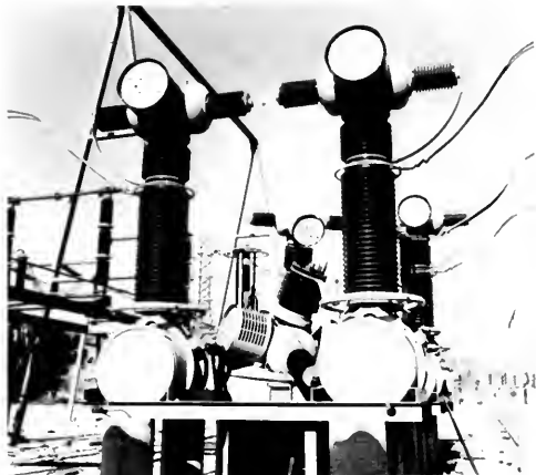
Photo 23. Sylmar Converter Station. Pneumatic circuit breakers. Two relatively undamaged units in foreground. Los Angeles Department of Water and Power photo.
